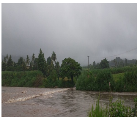
Figure 12d: Toge Crossing in Ba completely submerged. Source: Fiji Roads Authority.
