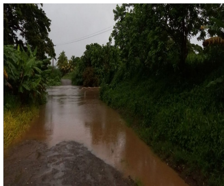
Figure 12a: Mate Crossing, Nadi, on the 6 th . Source: Fiji Roads Authority.
