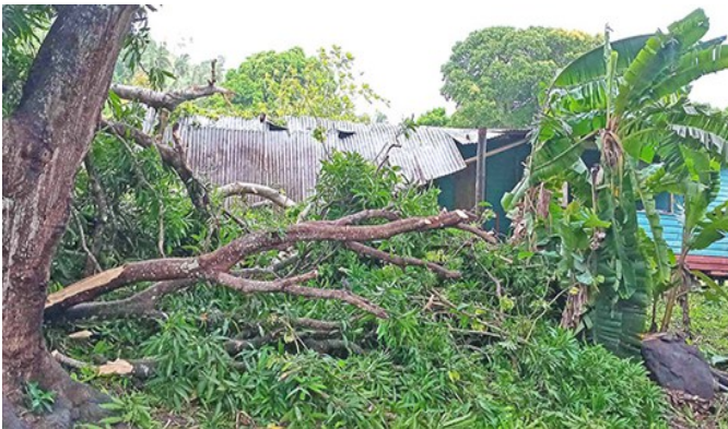
Figure 13e: A home in Cicia, Lau, partially damaged from fallen branches on the 25th . Source: Fiji Sun.
