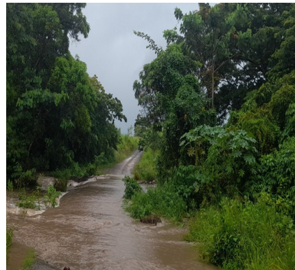
Figure 12f: Kabisi crossing, Sigatoka. Source: Fiji Roads Authority.
