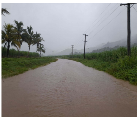
Figure 12g: Surface flooding in Namoli Rd, Labasa on the 28 th . Source: Fiji Roads Authority.
