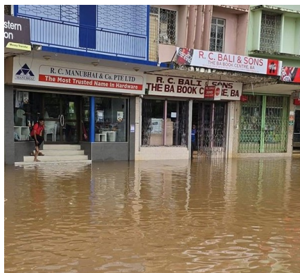
Figure 12h: Flooding of Ba town on the 31 st . Source: FijiVillage
